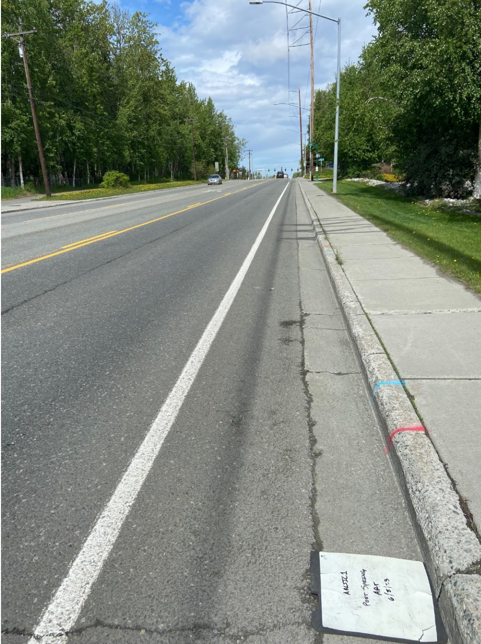
Figure 4-1 2023 ‘Visually Clean’ Photo Example (Post Spring Sweep ARDSA Arctic1)
